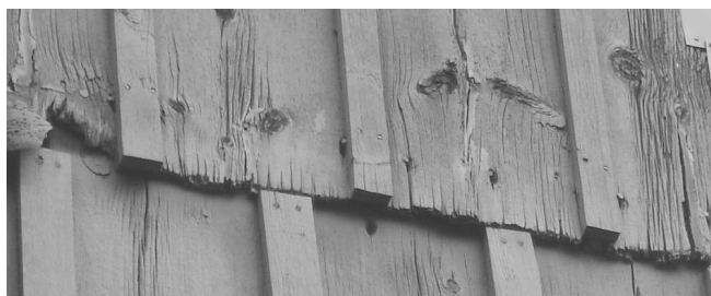
Barn siding to be replaced
